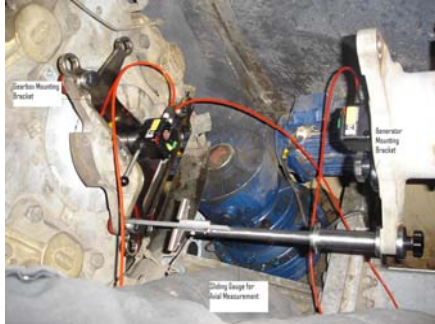
Fig. 3 – Alignment with coupler removed
